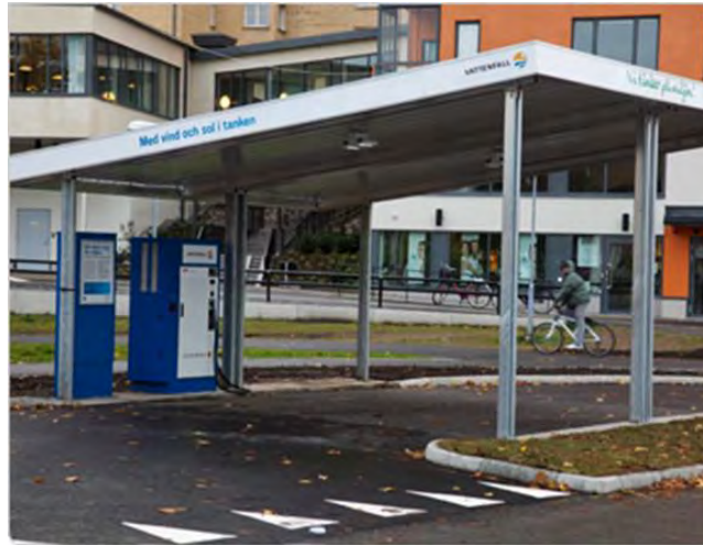
Figure 5 A Vattenfall fast charging station in Tyresö (Sweden) with a canopy and lighting. Photo: Elisabeth Redlig
